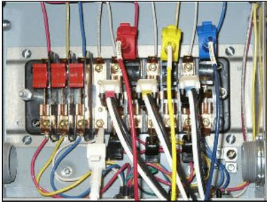
Insert direct current probes and move A, B, C voltage clips to top of currents. Connect white voltage clip to Neutral.
