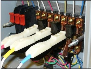
Insert direct current probes into test switch.
