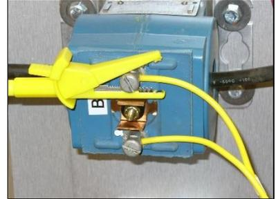
Connect the yellow (+) voltage cable connection to the CT secondary for B phase
