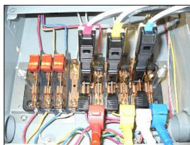
Move the white lead (Neutral) to the bottom of C phase current.
