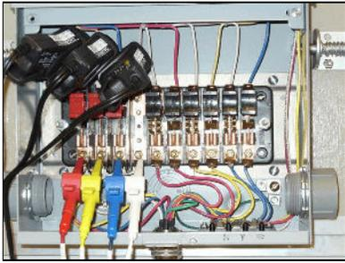
Clamp current probes around voltage wires at test switch. Connect voltage leads as normal.
