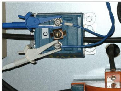
Connect the blue (+) and move the white (-) voltage cable connections to the CT secondary for C phase
