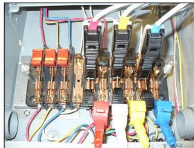
Move the white lead (Neutral) to the bottom of B phase current.
