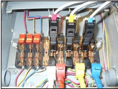
Insert direct current probes into test switch. Move the voltage leads to the bottom of the currents. Connect the white lead (Neutral) to the bottom of A phase current.
