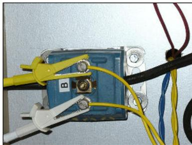
Connect the yellow (+) and move the white (-) voltage cable connections to the CT secondary for B phase
