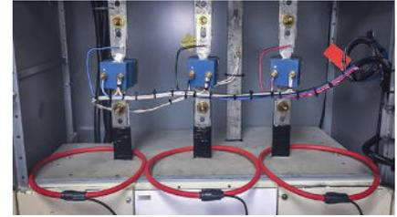
Wrap or connect primary probes around conductors at CT
