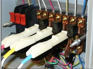
Insert direct current probes into test switch.
