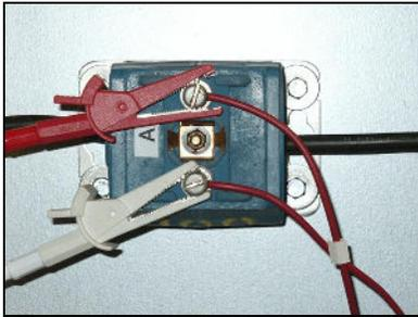
Connect the red (+) and white (-) voltage cable connections to the CT secondary for A phase
